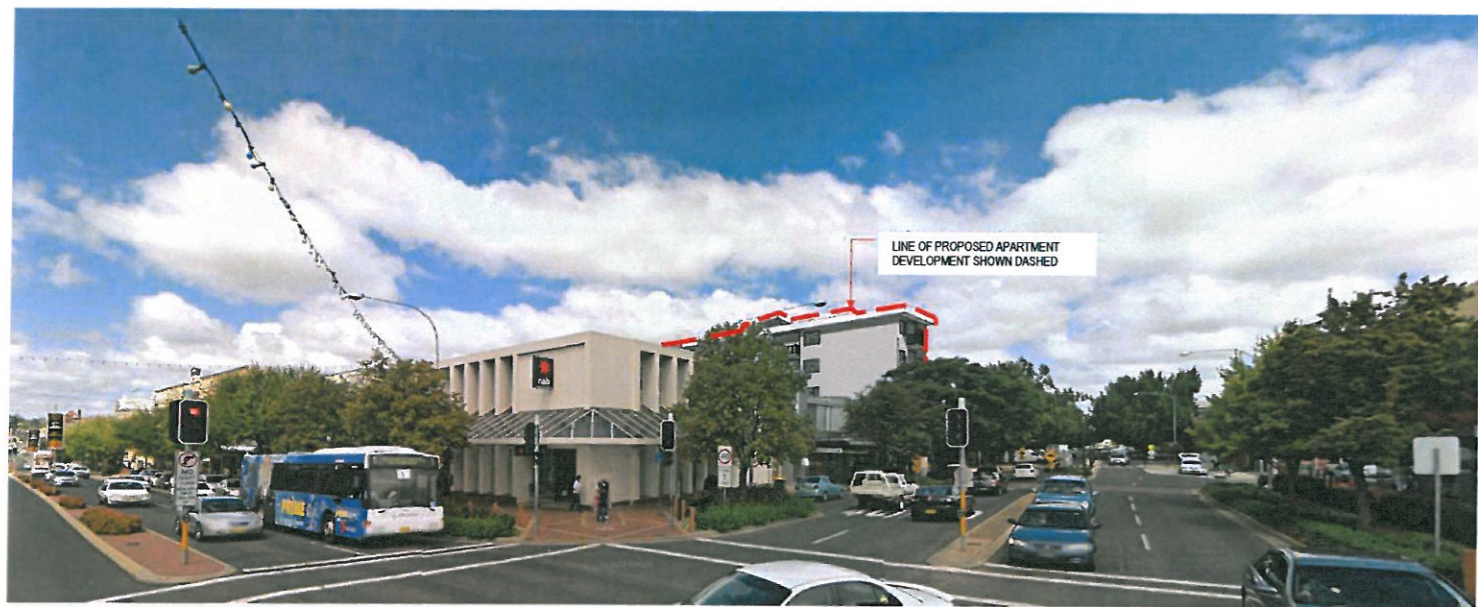
IMAGE 1 - INDICATIVE VIEW FROM SUMMER STREET TOWARDS ANSON STREET AND PROPOSED APARTMENT DEVELOPMENT
